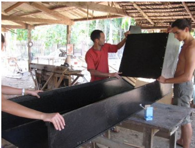
Figure 7.63: Fixing the parts of the dryer
