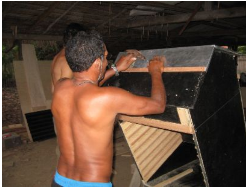
Figure 7.64: Covering the roof with an aluminum panel
