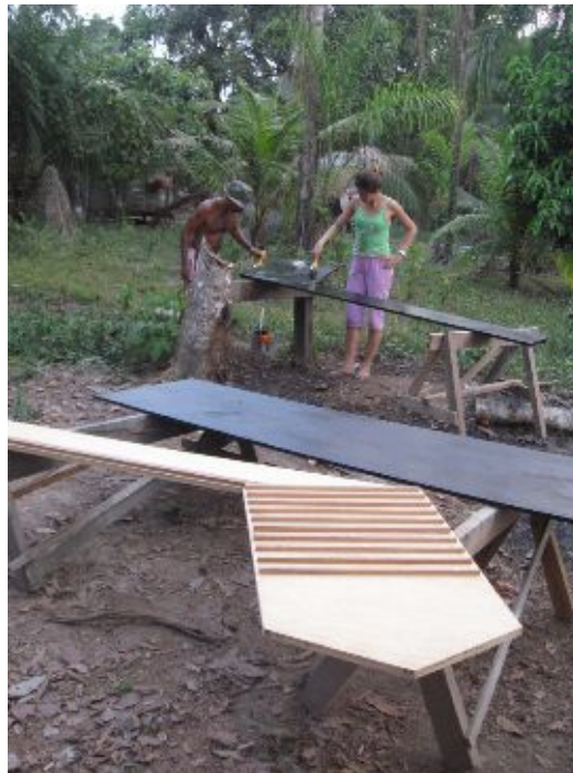
Figure 7.60: Painting all the parts of the dryer
