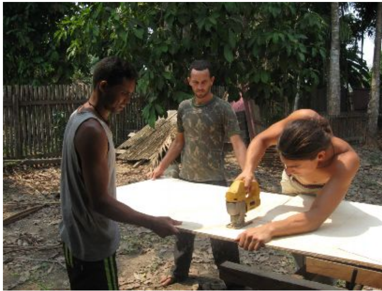
Figure 7.58: Sawing of plywood
